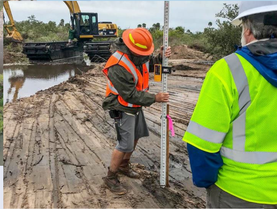
Leveling restored areas
